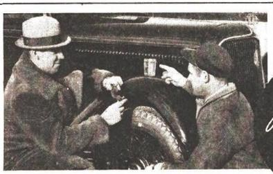
A PRACTICAL TEST of Floating Power. The engine is racing, but the glass of water does not tremble. Suspending the motor in balance is the secret.
